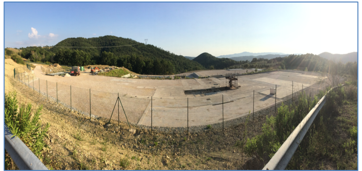
Figure 4 – Drilling Pad completed
